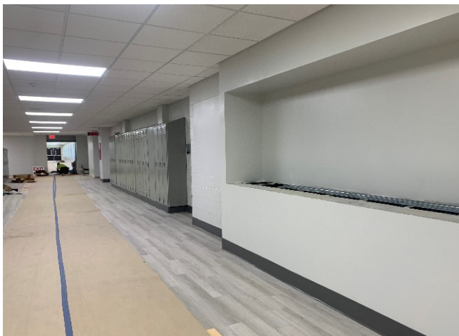
CES - corridor flooring installation
