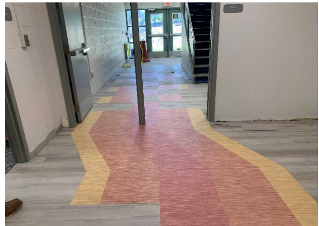
CES - corridor flooring installation
