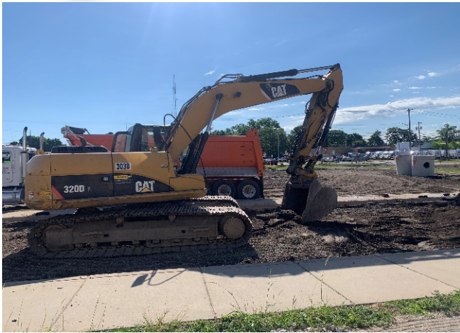
CES - Parking Lot Demolition
