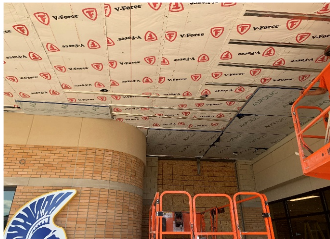
CES - exterior metal panels installation
