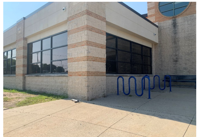
CHS - Window replacement at High School
