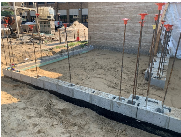
CES - Gym Expansion CMU Walls
