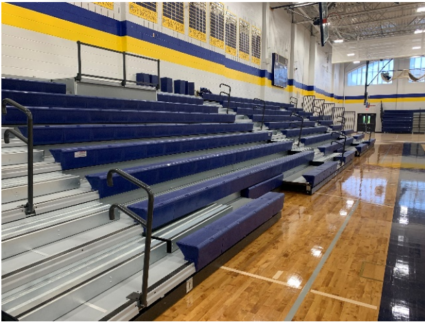
CHS - Main Gym Bleachers installation
