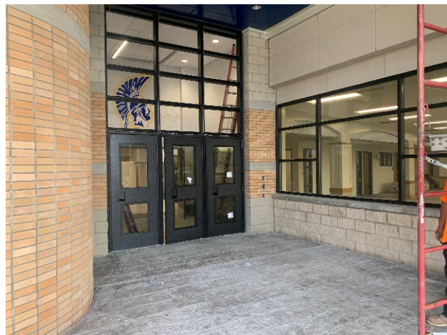
CES - Storefront doors installation at Main Entrance
