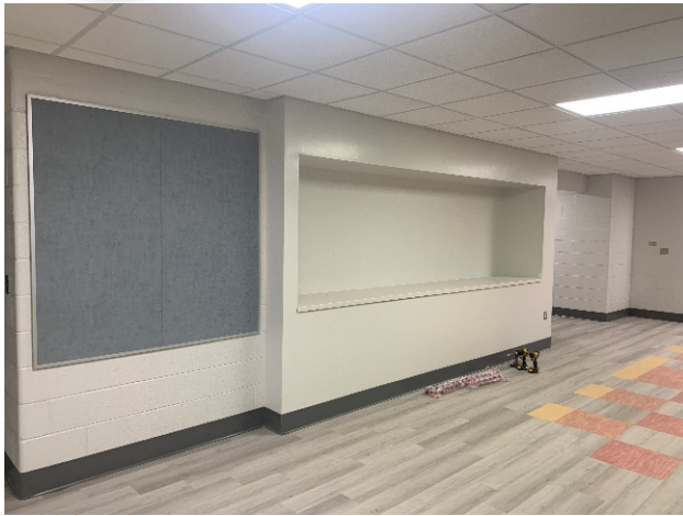
CES - Corridor Tackboards and Display Cases
