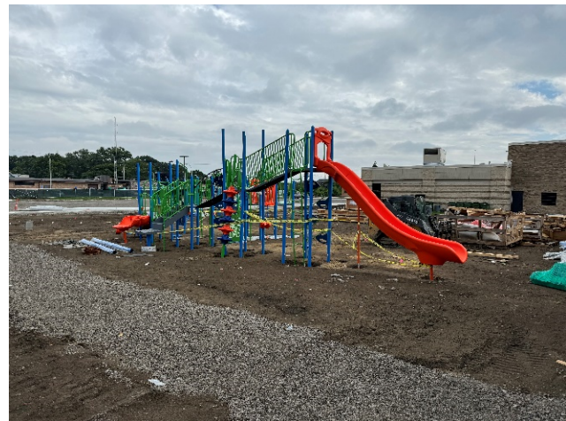
CES – Playground Installation – In Progress
