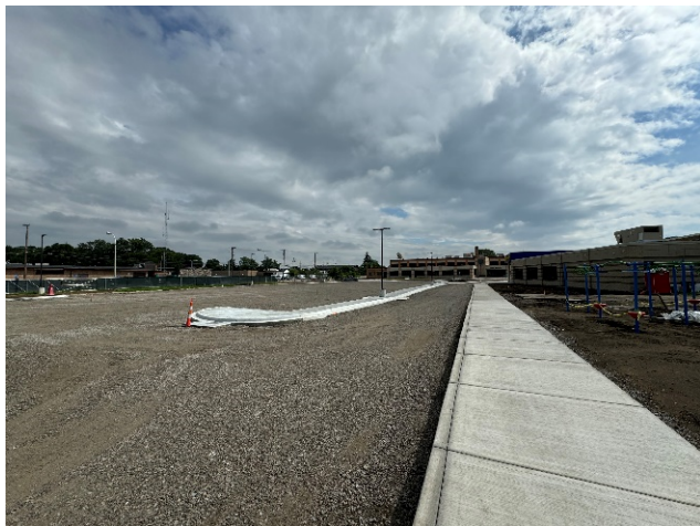
CES/CHS – Parking Lot – Ready for Asphalt
