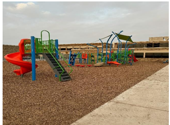
CES – Playground Installation – Complete
