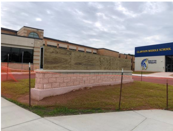
Clawson Schools – Monument Sign In Progress
