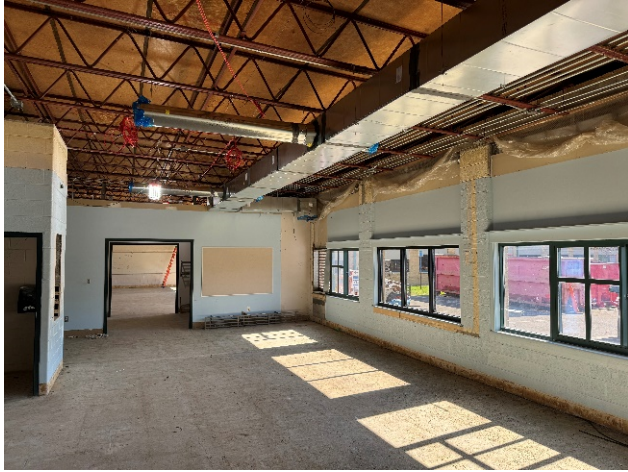
ECC – OH Mechanical Install & Window Install
