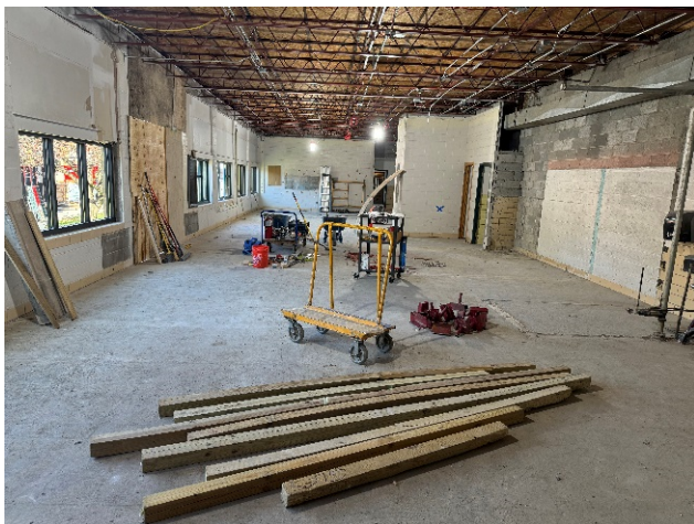
ECC – Demolition and Prep for New Main Office
