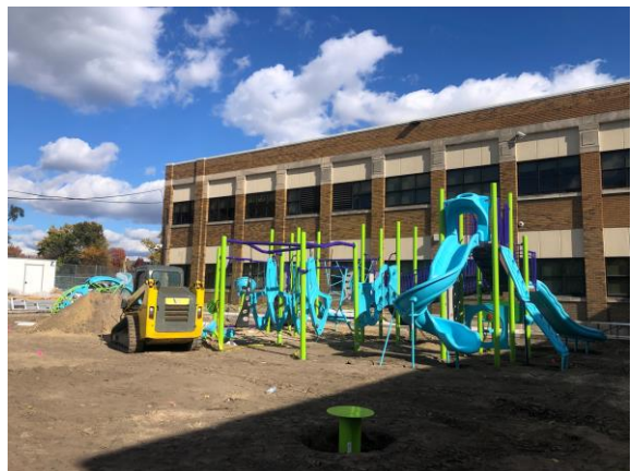
CES – Playground In Progress
