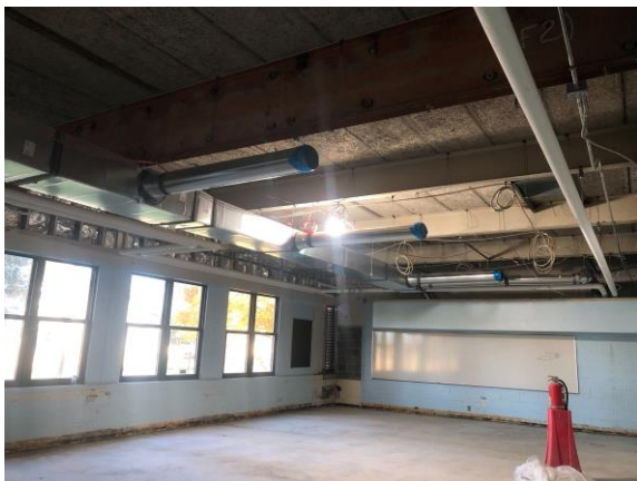
ECC – OH Mechanical Install In Progress
