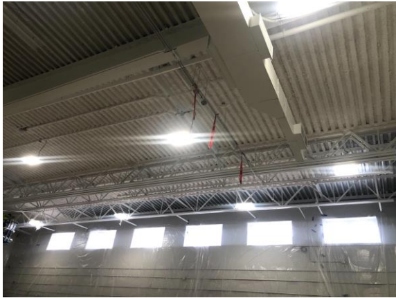
CES – Gym Addition K13 Acoustical Spray In Progress
