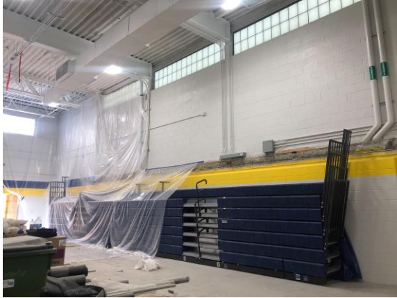
CES – Gym Addition Bleachers & Painting In Progress
