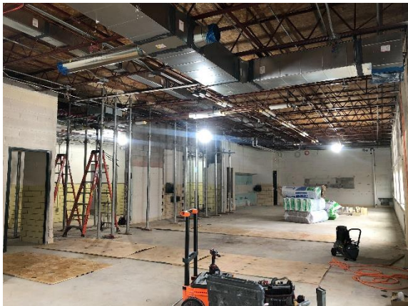
ECC – Overhead Electrical Install In Progress
