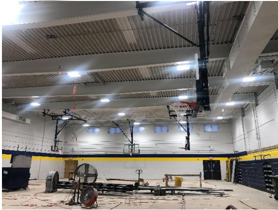
CES – Gym Addition Basketball Hoops In Progress
