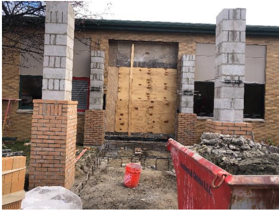
ECC – Future Main Entrance In Progress
