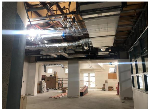
ECC – Library MEP In Progress
