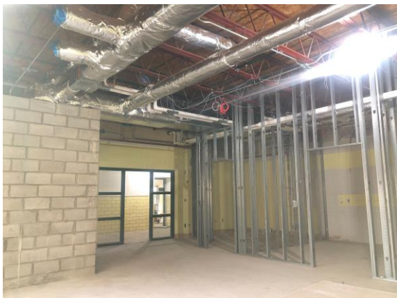
ECC – Office Space In Progress
