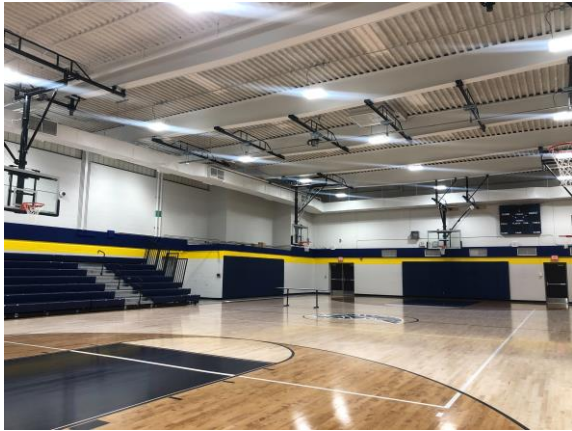
CES – Gym Addition Complete
