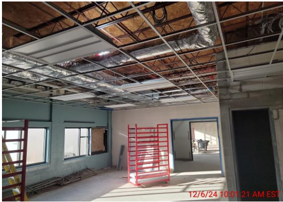
ECC – Interior Ceiling Grid & Lighting In Progress
