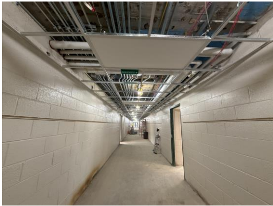
ECC – Corridor Interior Ceiling Grid & Lighting In Progress
