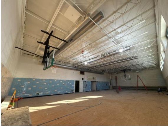
ECC – Gym HVAC Duct In Progress
