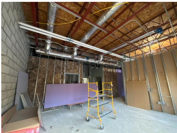
ECC – Future Main Office Wall Insulation & Board In Progress
