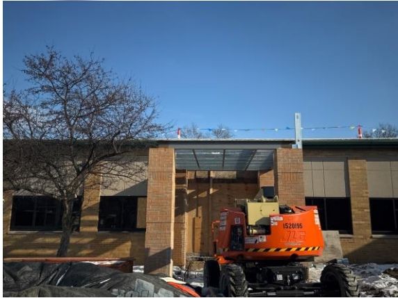
ECC – Main Entrance Canopy Framing In Progress
