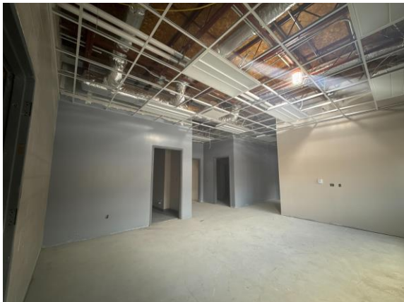
ECC – Main Office Ceiling & Painting In Progress
