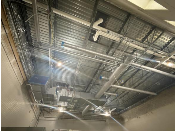
ECC – Cafeteria Ceiling MEP In Progress
