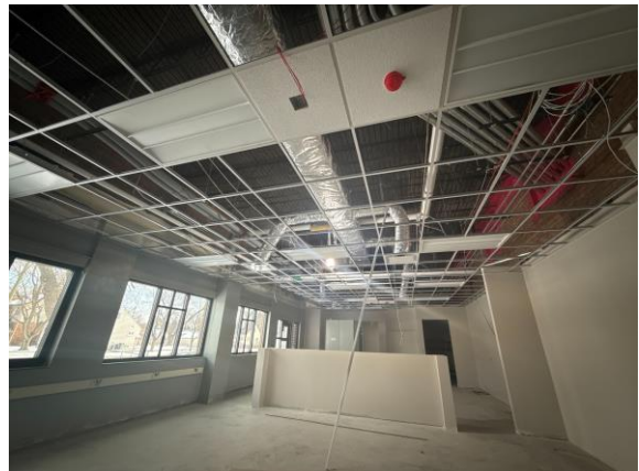
ECC – Smoke Detector Install In Rooms & Corridors In Progress
