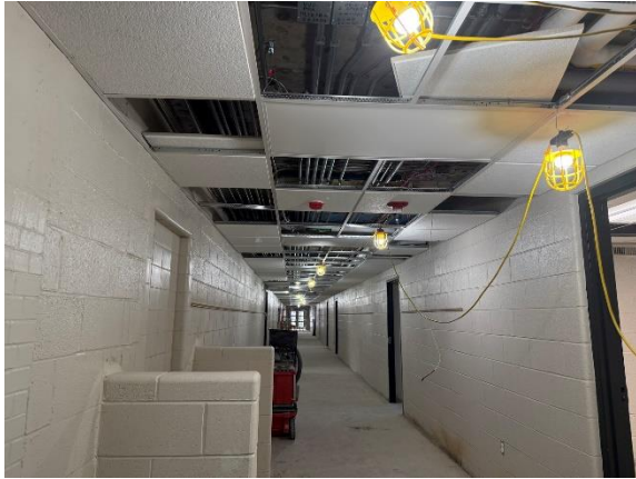
ECC – Corridor Ceiling In Progress
