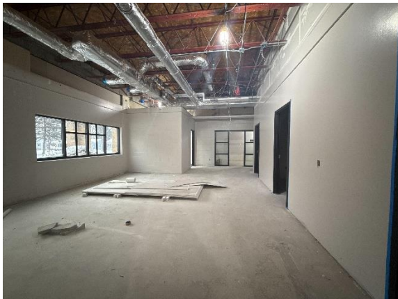
ECC – Office Space In Progress
