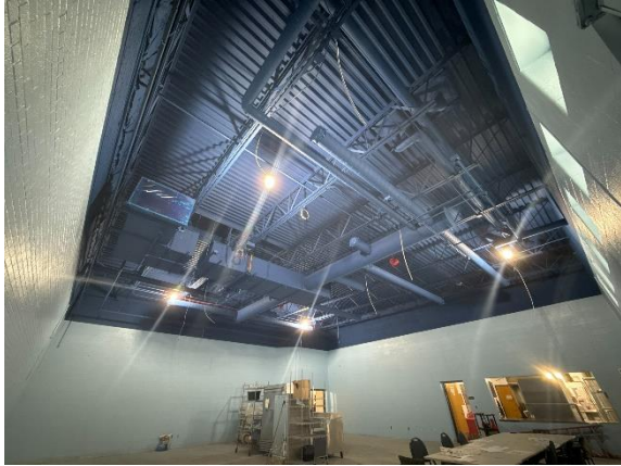
ECC – Cafeteria Painting In Progress
