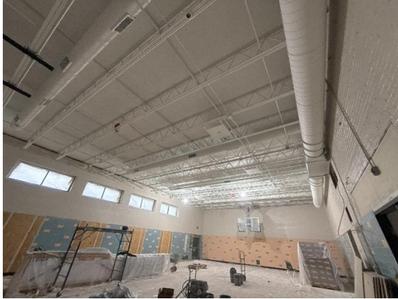
ECC – Gymnasium Paint In Progress
