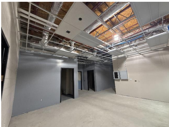
ECC – Main Office Space In Progress
