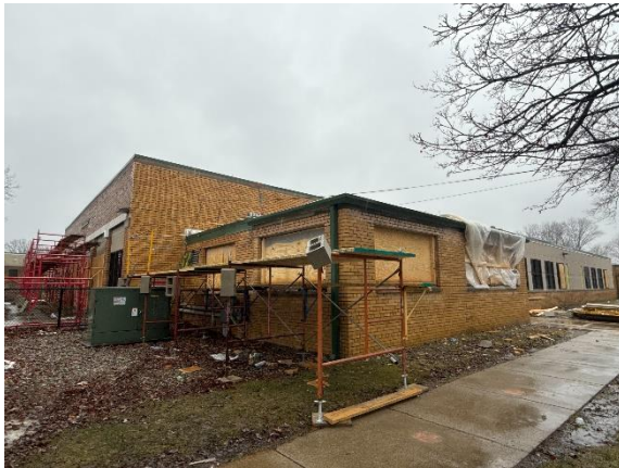
ECC – North Side Exterior Lentils In Progress
